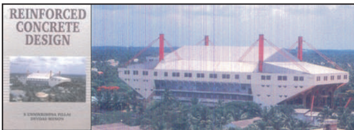
Structural design of a unique ship-shaped indoor GCDA stadium for the Regional Sports Centre, Kochi (1993)
