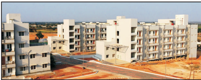
GFRG hostel buildings at IIT Tirupati
