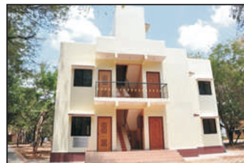
GFRG demo building at IIT Madras
